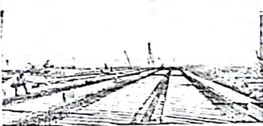
DECK SHEET LAYING FOR DECK SLAB
